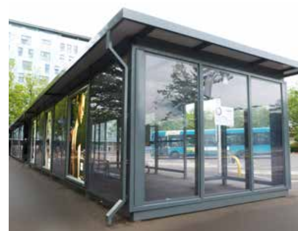
MK Station Shelter
